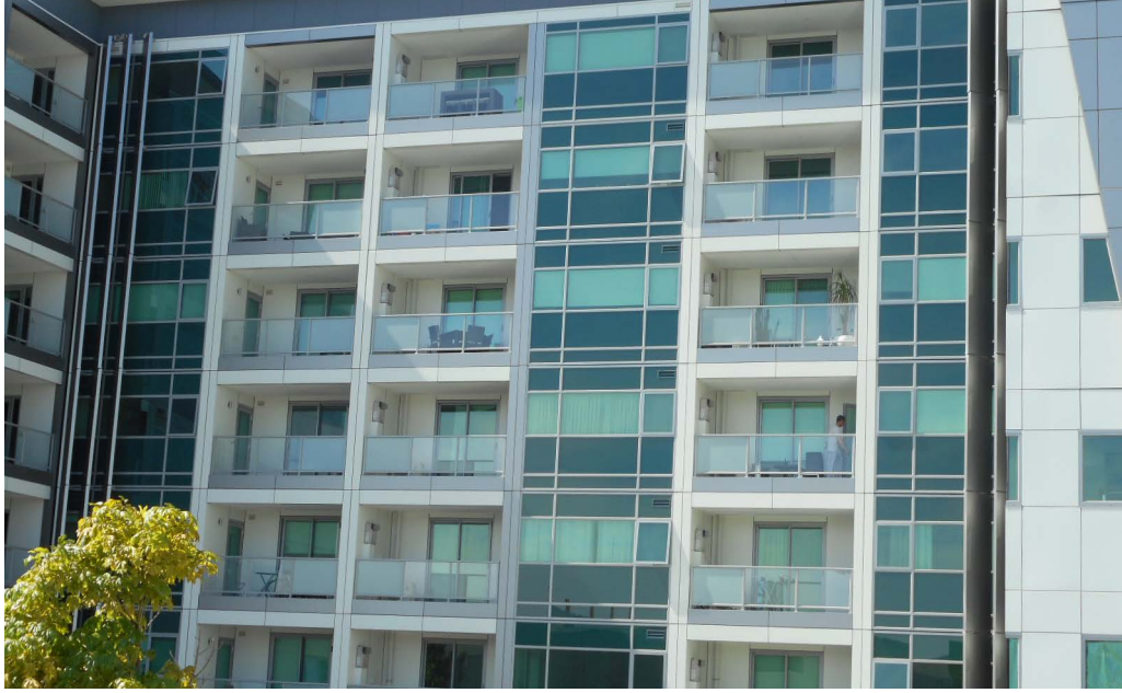
Complying flues with sideways draft diverters
