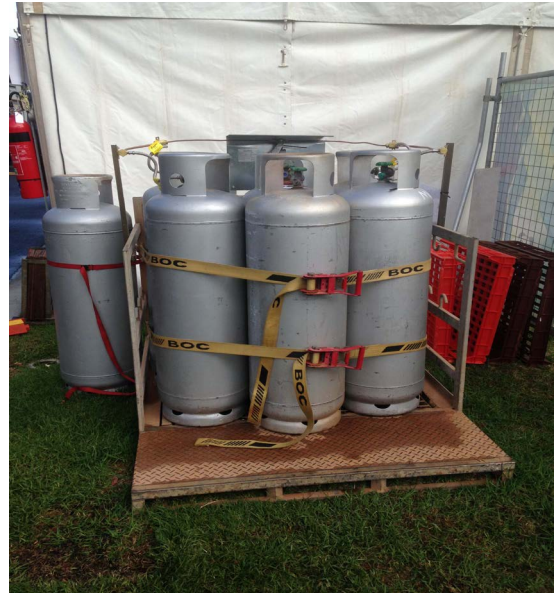
Bank of four 45Kg LP Gas cylinders secured and caged
