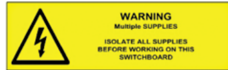
Figure 4: Typical warning label
