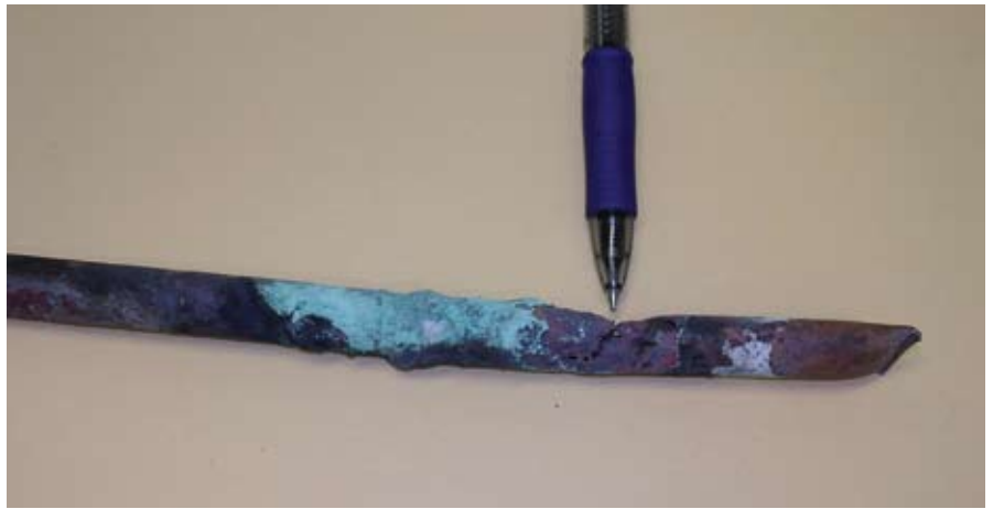
Corroded copper pipe
